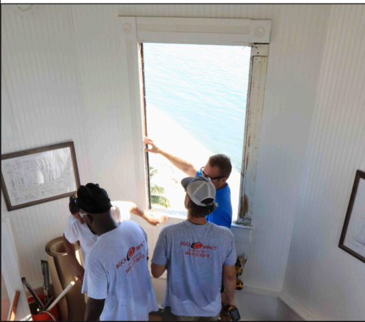
SERVICE ROOM WINDOW PREP CIRCA AUG 2023
