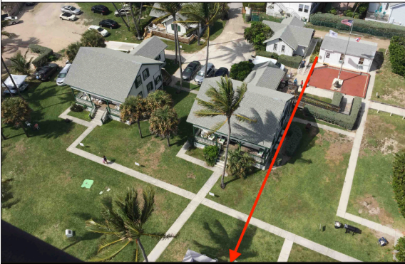
UNDERGROUND FIBER OPTIC CONDUIT PATH FROM GENERATOR ROOM TO BASE OF LIGHTHOUSE CIRCA 2023
