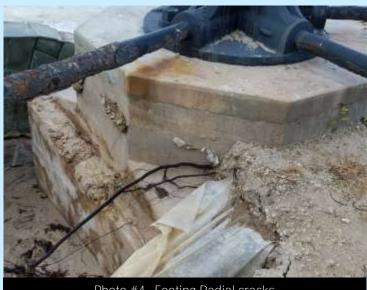
Photo #4—Footing Radial cracks Art Makenian
