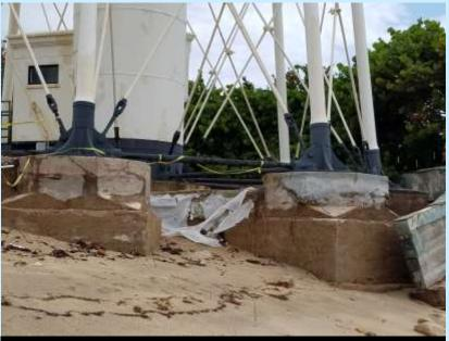
Photo #3 - Lighthouse Foundations Exposed Art Makenian
